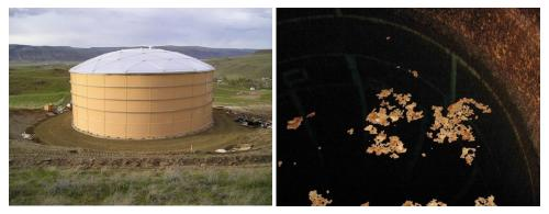
Stagnant water tends to stratify in layers of different temperatures. The topmost layer is warmest, encouraging bacterial growth and nitrification. The bacterial growth in water tank on the right is indicative of undertreated water.
